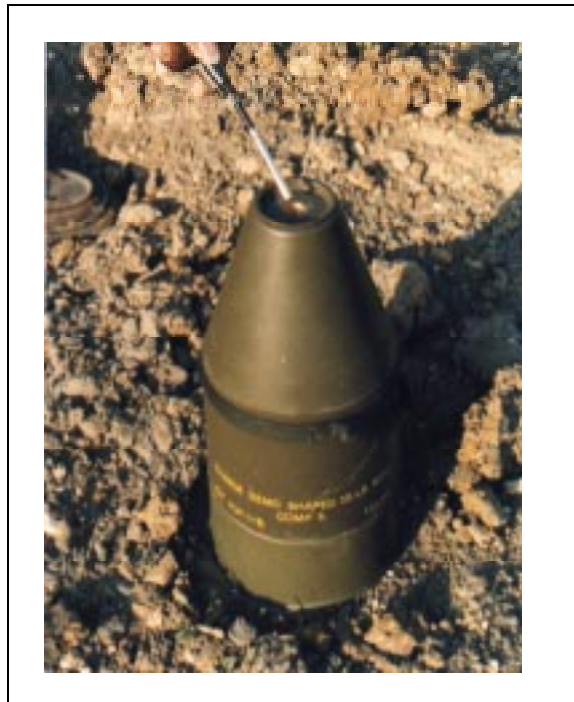
Figure 7-10. Priming shaped charges with MDI
